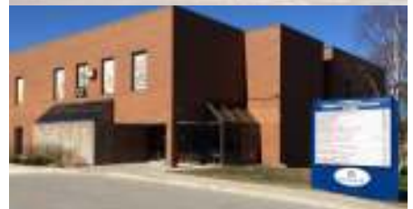
Alliston in 1891, after the fire that destroyed the town (top), Windsor House today (middle), Orangeville Medical & Professional bldg.(today).
